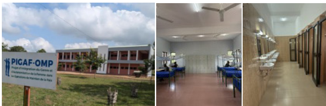
30-bed accommodation facility for women, Centre National d'Instruction, Kara, Togo, June 2025.
